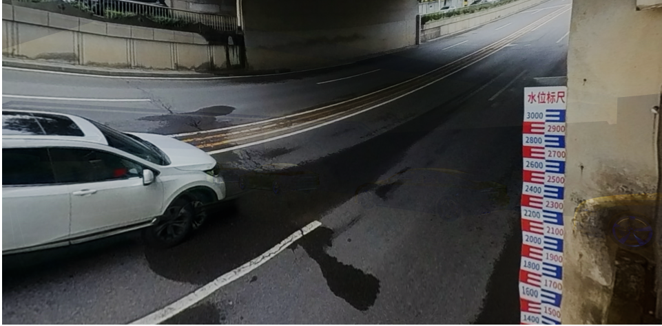
Figure 2: Field Observation of the Flood-prone Areas
